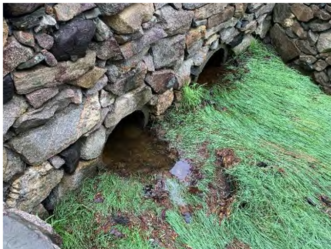
4 Brickyard Circle – 1 (Drainage Course)
