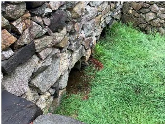
4 Brickyard Circle – 1 (Drainage Course)
