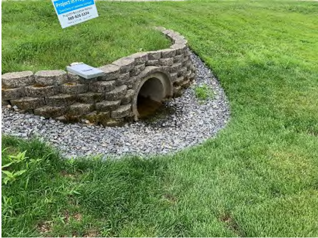
29 Gundalow - 1 (Drainage Area)
