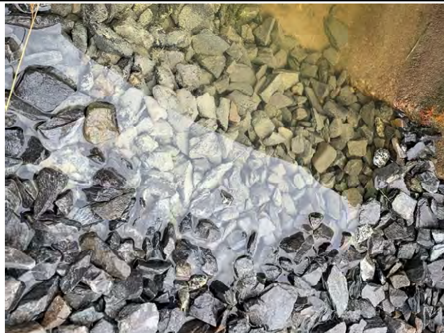
29 Gundalow -1 (Drainage Area)
