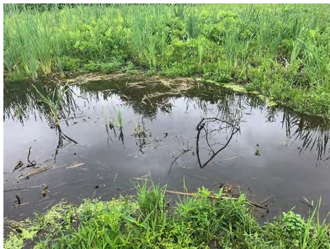
Knight's Brook – 3 (Above Duct Bank in Brook)
