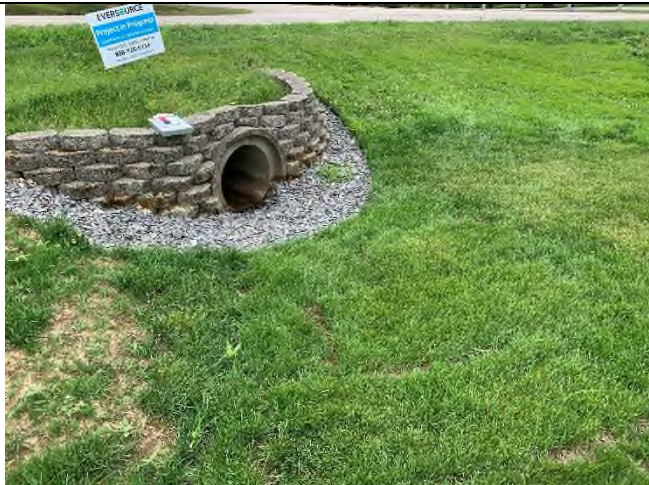
29 Gundalow -1 (Drainage Area)
