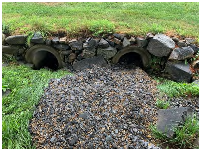
64 Gundalow – 2 (Drainage Course) with stone deposition
