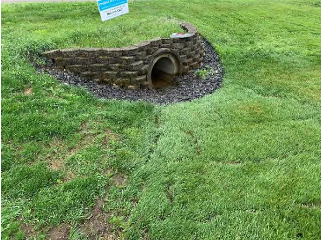
29 Gundalow -1 (Drainage Area)
