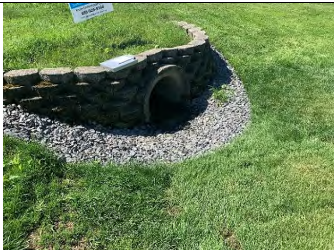
29 Gundalow - 1 (Drainage Area)
