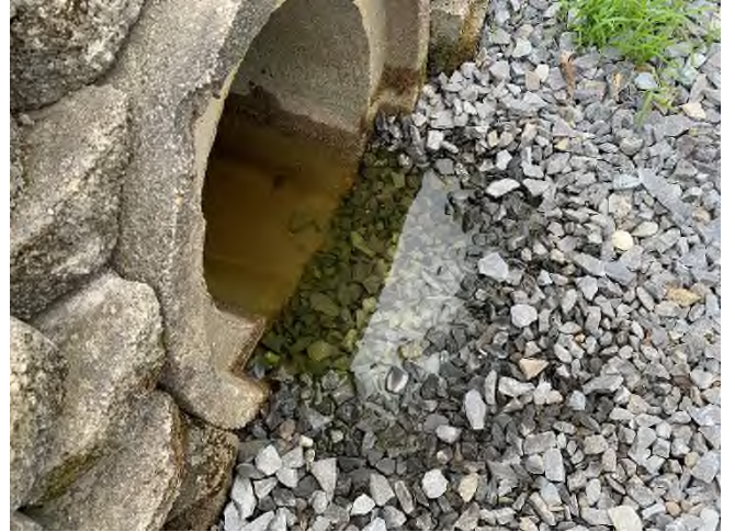
29 Gundalow - 1 (Drainage Area)
