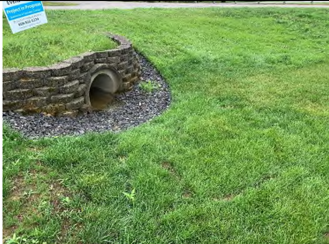
29 Gundalow -1 (Drainage Area)
