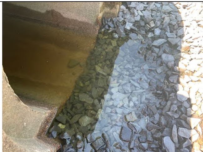
29 Gundalow - 1 (Drainage Area)
